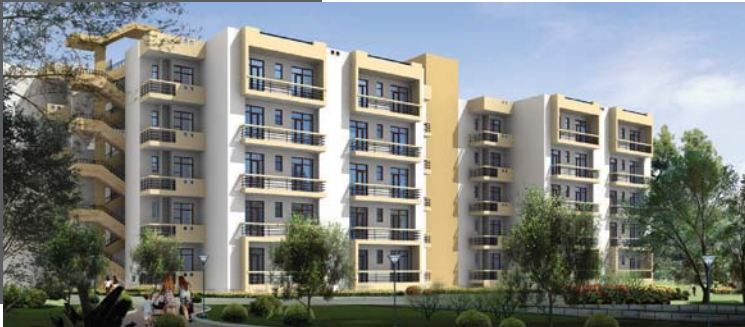
M/S CHANDERLEKHA INFRASTRUCTURE (P) LTD. MATHURA
